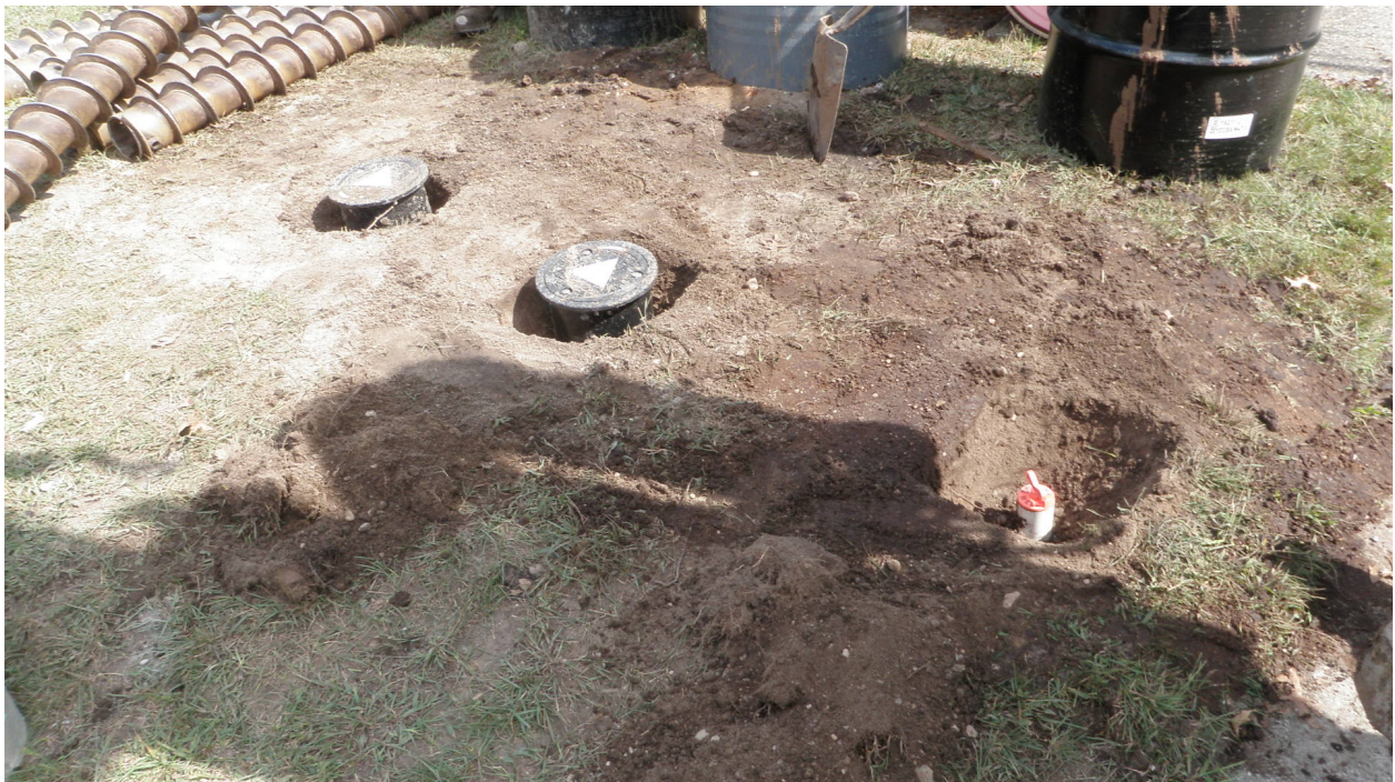
Oxygen injection well installation at 87 Community Road
