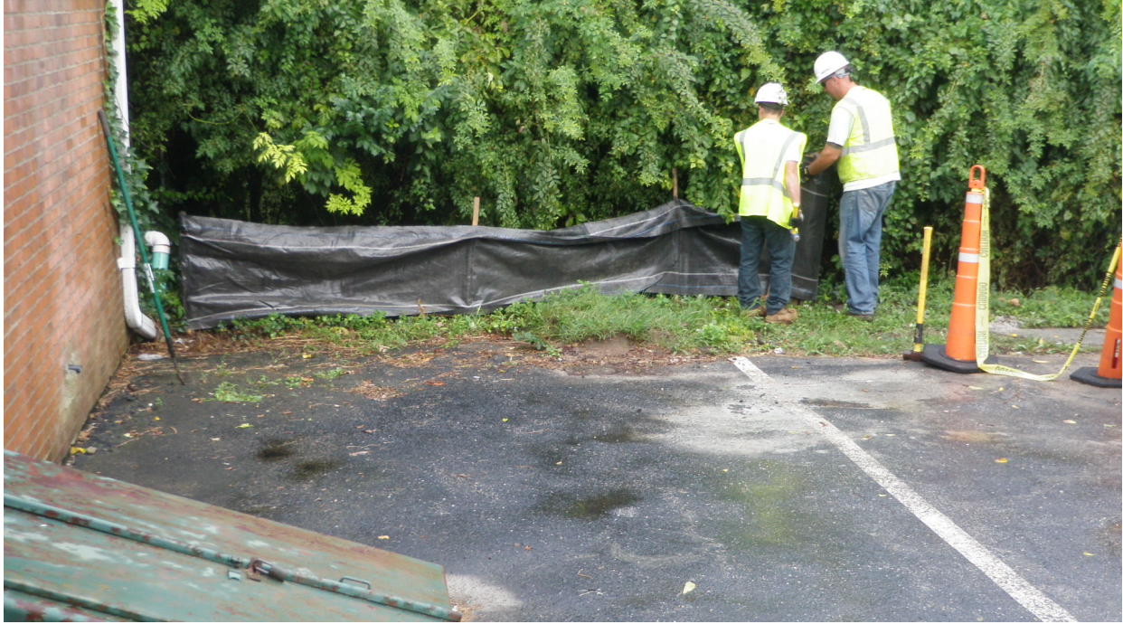
National Grid's contractor, EnviroTrac, installing silt fence at 87 Community Road
